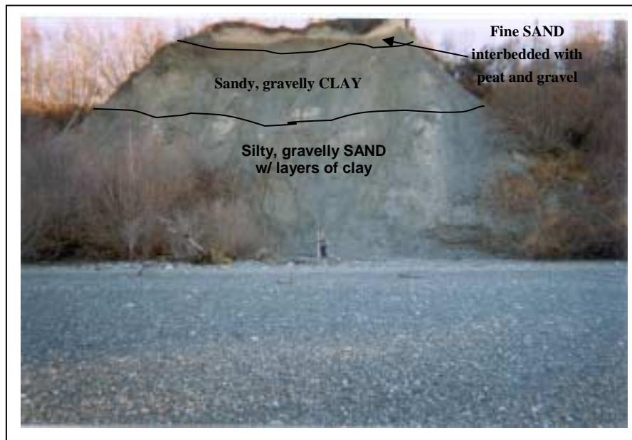
Photograph A-2: East bluff near Boring A-12 (note person in middle for scale).
